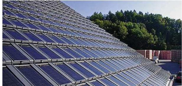
**Abb. 3.3.1/6:** Solardachziegel (Quelle: [www.realize-energysystems.com](http://www.realize-energysystems.com))
